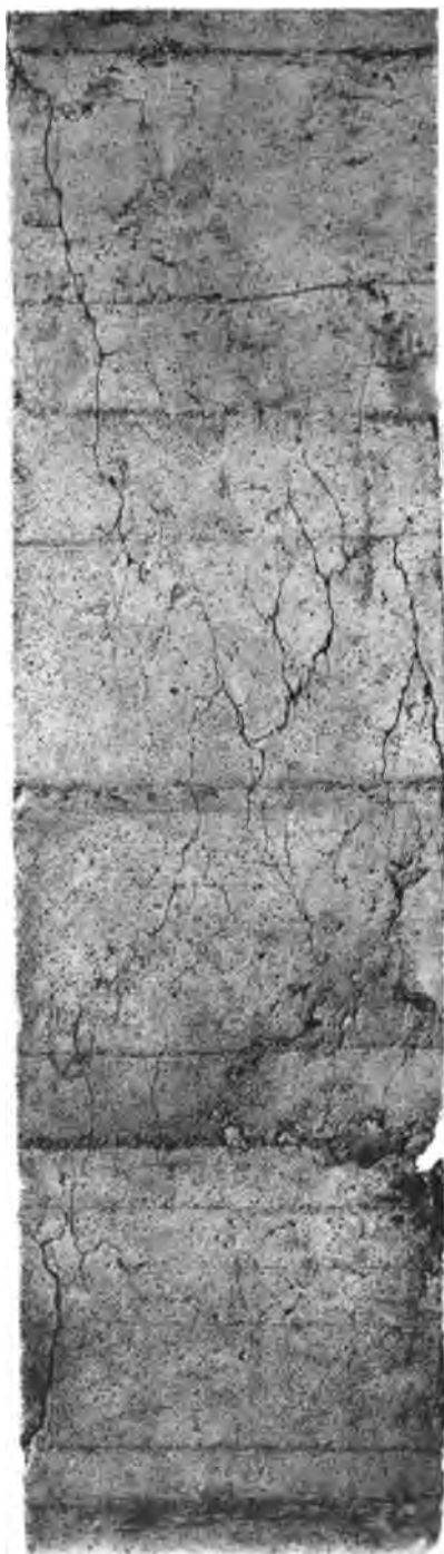
CONCRETE COLUMN NO. 1493. APPEARANCE AFTER TESTING. MIDDLE PART OF ITS HEIGHT.
